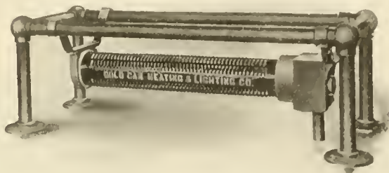
ELECTRIC HEATER IN PLACE.
